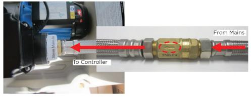
**Step 8:** Install isolation valve and pressure limiting valve to the mains inlet line.
