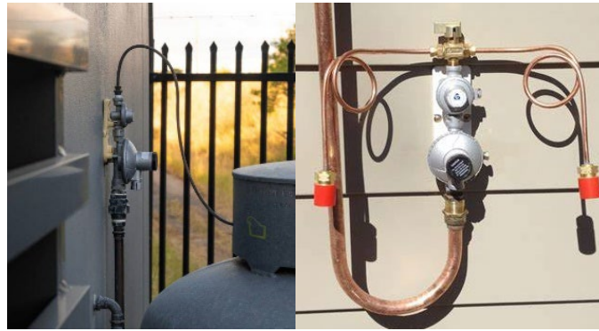
Figure 1. a) 1 cylinder and pigtail connected into top of regulator. b) 2 pigtails connected via manual changeover valve
